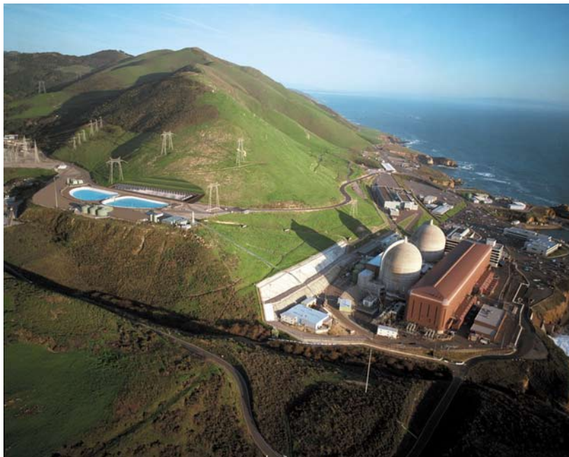
Diablo Canyon Nuclear Power Plant - California
